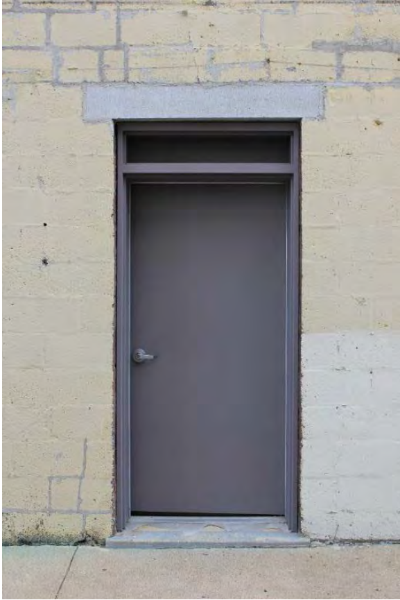
Figure 3.328, Old Jail, west elevation, view of north door.
