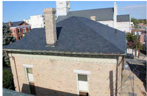
Figure 3.239, Wallace Library, South elevation, detail of roof.
