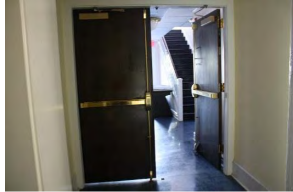
Figure 3.108, Historic Courthouse, First Floor, Room 130, view looking north at hollow-core double doors.
