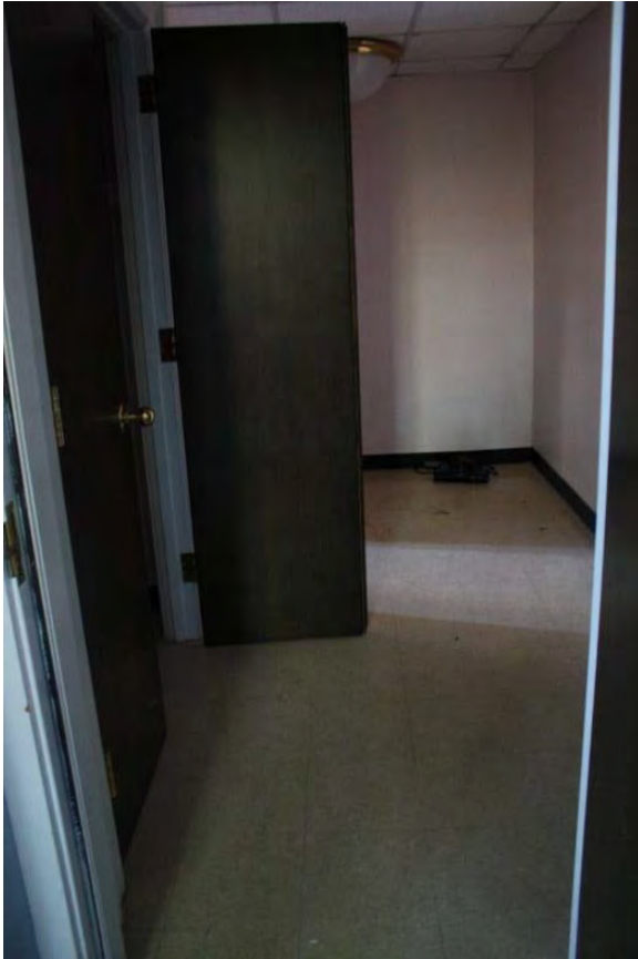
Figure 3.161, Historic Courthouse, Second Floor, Room 213, general view looking east.
