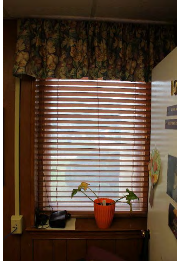
Figure 3.265, Old Wallace Library, First Floor, Room 101, view of typical first-story window. Note that first-story windows are the lower sections of double-height windows.
