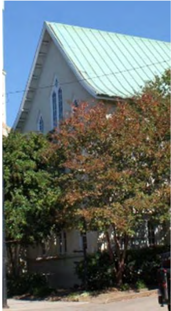
Figure 1.8, Fredericksburg Courthouse, South Wing, Existing roof. Photograph 2015.
