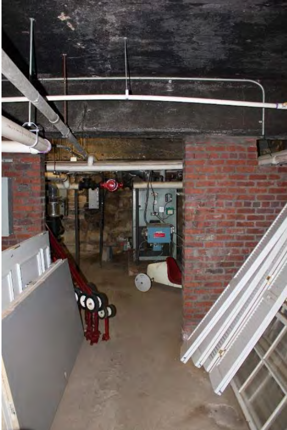
Figure 3.364, Old Jail, Basement, Room 003, general view looking south.
