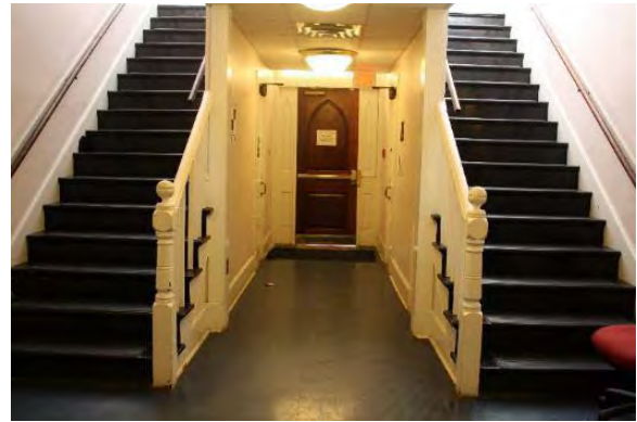
Figure 3.46, Historic Courthouse, First Floor, Room 101, overall view of stairway.
