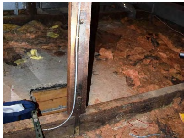
Figure 4.13: North wing roof king post tension strap
