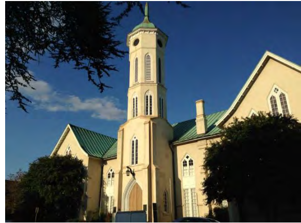
Figure 4.02: Main Façade (West Elevation) of Renwick Courthouse.
