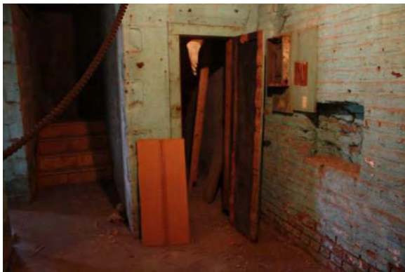
Figure 3.371, Old Jail, Basement, Room 004, general view looking east toward the stair.
