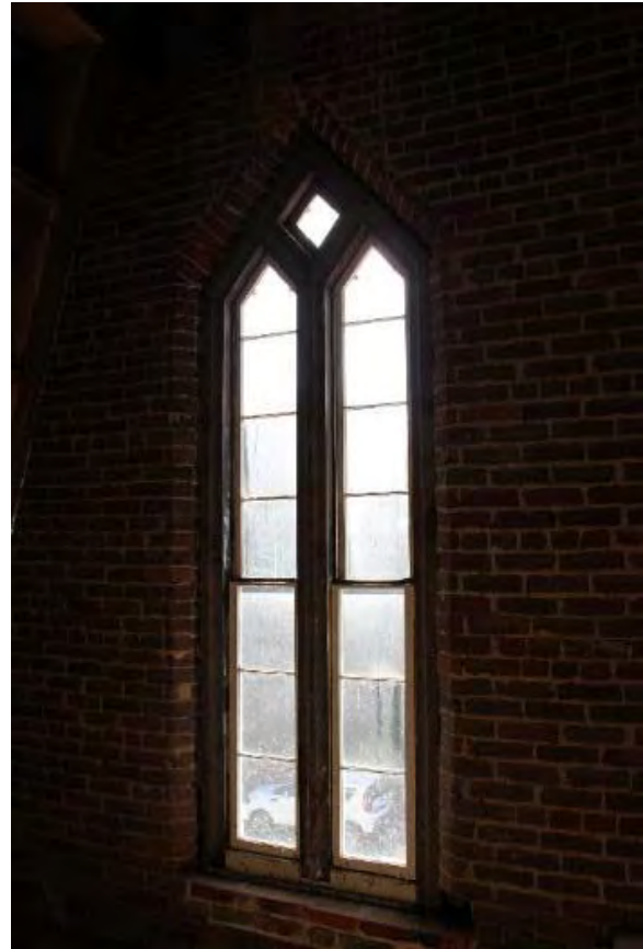
Figure 3.202, Historic Courthouse, Bell Tower, Room 302, view of a second-story window.
