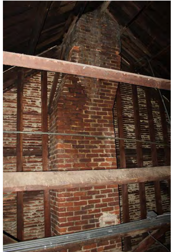
Figure 3.210, Historic Courthouse, North Attic, Room 303, view of chimney at south wall.
