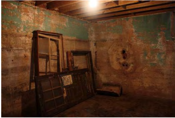
Figure 3.376, Old Jail, Basement, Room 005, general view looking northwest.
