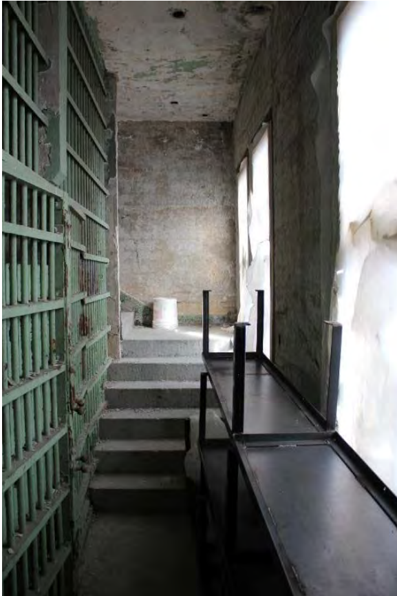
Figure 3.420, Old Jail, First Floor, Room 108, general view looking north.
