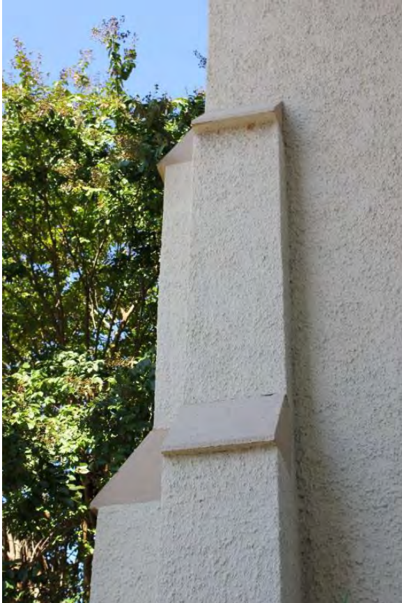
Figure 3.20, Historic Renwick Courthouse, north elevation, view of stucco buttresses.
