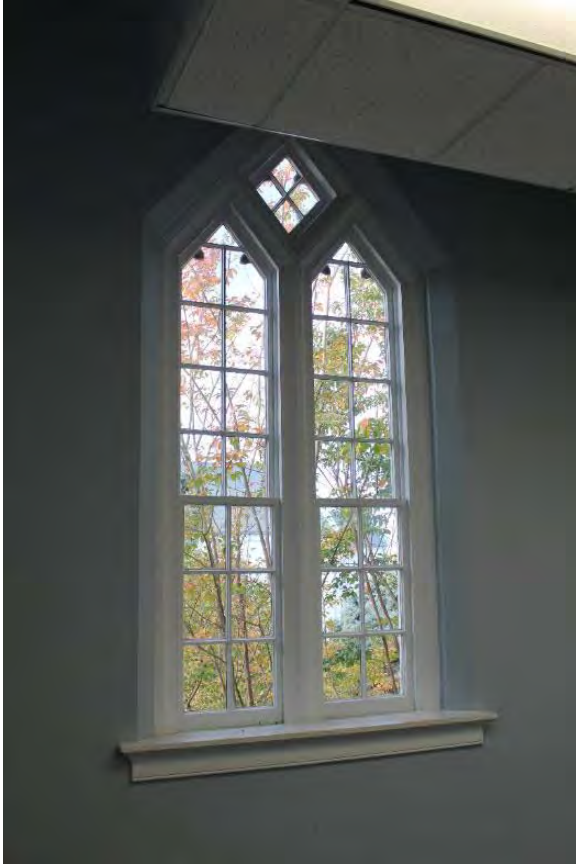
Figure 3.169, Historic Courthouse, Second Floor, Room 216, view of window at north wall.
