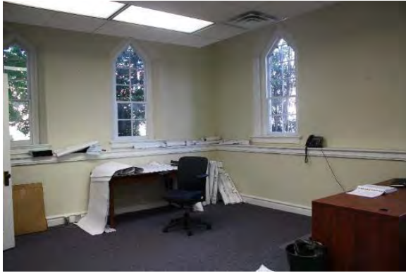
Figure 3.90, Historic Courthouse, First Floor, Room 123, general view looking northwest. Note the carpeted floor and the higher level of detail including molded chair rail and base.
