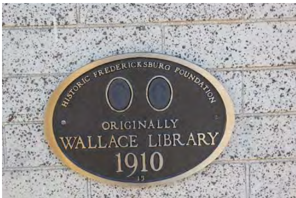
Figure 3.221, Wallace Library, West elevation, detail of Historic Fredericksburg Foundation plaque.
