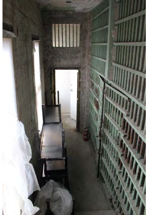
Figure 3.421, Old Jail, First Floor, Room 108, general view looking south.
