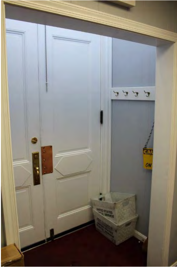
Figure 3.266, Old Wallace Library, First Floor, Room 102, general view looking west. Note the early-twentieth-century paneled wood exterior doors.
