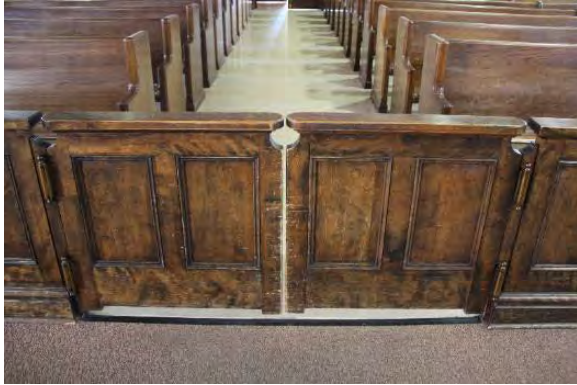
Figure 3.159, Historic Courthouse, Second Floor, Room 212, view of the swinging doors at the bar. Note the heavy wear and scratching where the doors meet.
