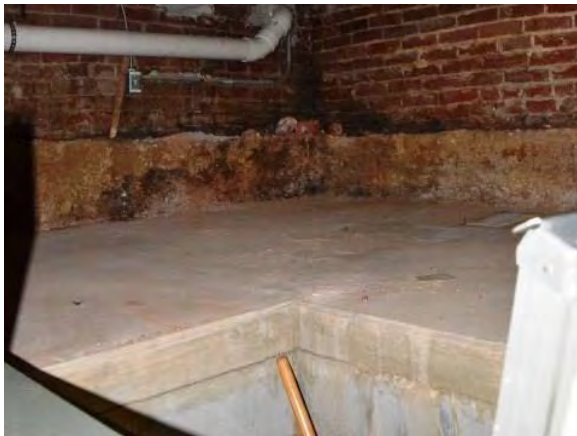
Figure 4.56: Concrete underpinning haunch in west half of basement
