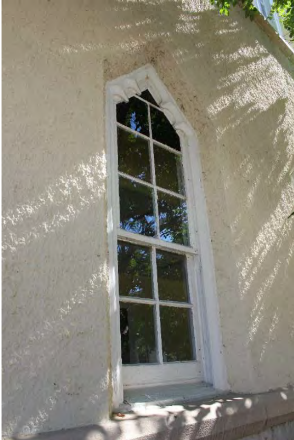
Figure 3.10, Historic Renwick Courthouse, west elevation, detail view of a first-story window.
