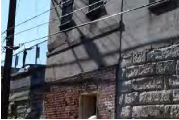
Figure 4.66: Southern section first floor slab edge visible from exterior
