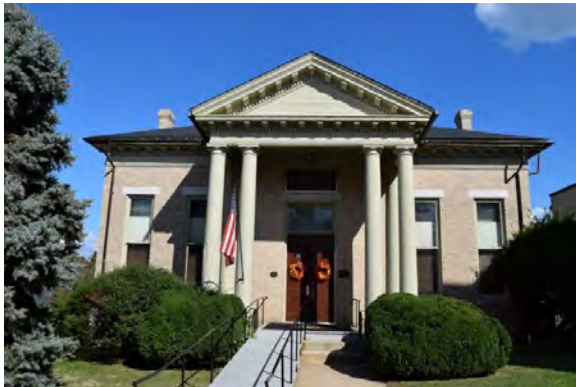
Figure 4.03: Main Façade (West Elevation) of the Fredericksburg Historic Library.
