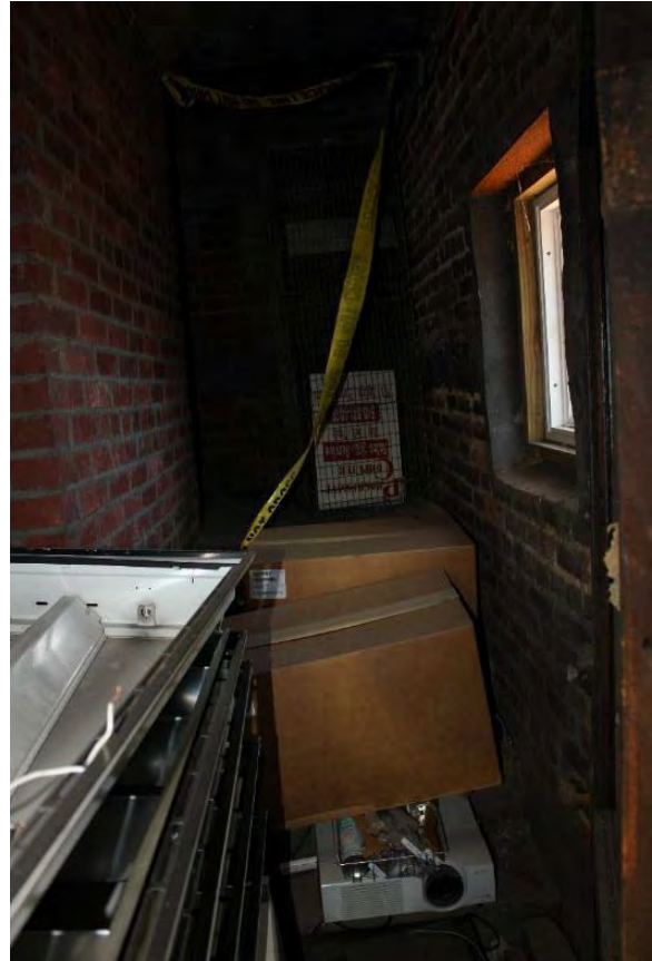
Figure 3.363, Old Jail, Basement, Room 003, general view looking north in the hall at the east wall. Note the stored material making it difficult to access all parts of the room.
