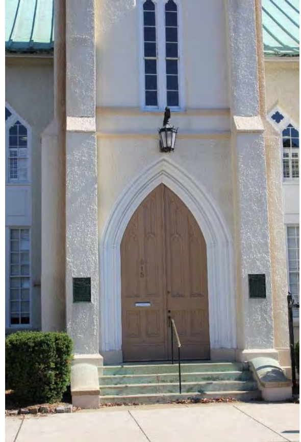
Figure 3.4, Historic Renwick Courthouse, west elevation, view of first story of bell tower, including entry doors.
