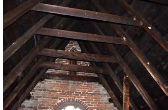
Figure 4.39: South wing stair hall roof framing
