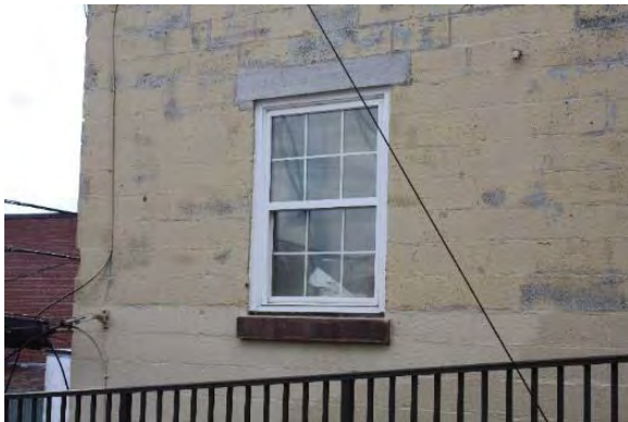
Figure 3.333, Old Jail, north elevation, view of first-story window.
