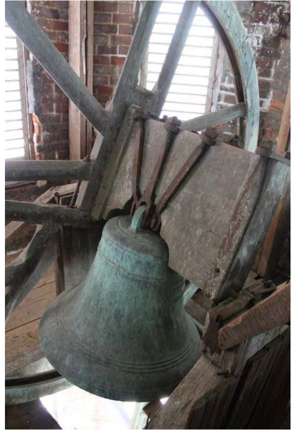
Figure 3.205, Historic Courthouse, Bell Tower, Room 302, view of Revere bell.
