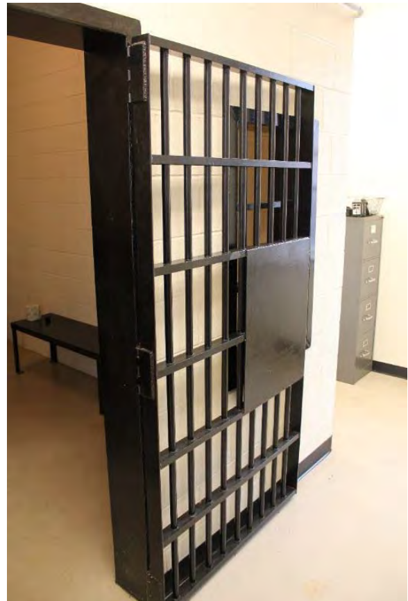
Figure 3.397, Old Jail, First Floor, Room 103, view of the jail cell door.
