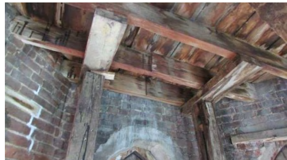
Figure 20: Bell floor framing existing showing
