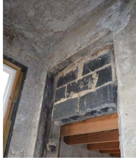
Figure 4.82: Second floor doorway between center building and northern addition
