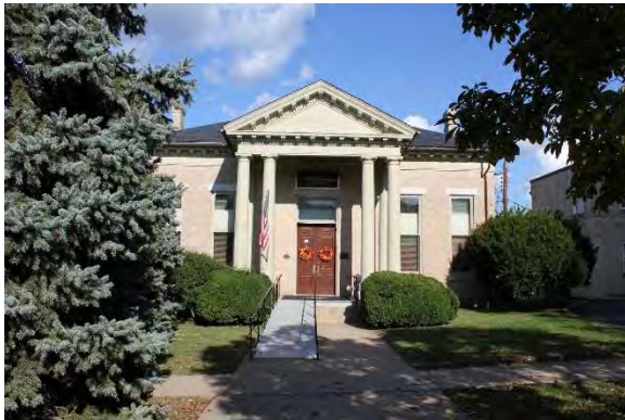
Figure 1.13, Wallace Library. Note the building's excellent exterior physical integrity. Photograph 2015.
