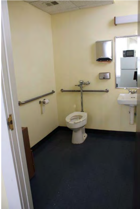
Figure 3.64, Historic Courthouse, First Floor, Room 114, general view looking north.
