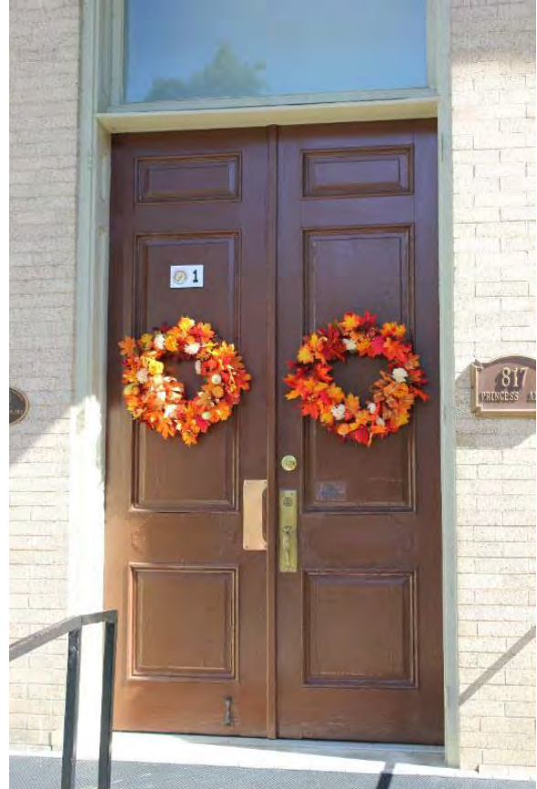
Figure 3.216, Wallace Library, West elevation, detail of double entry door.
