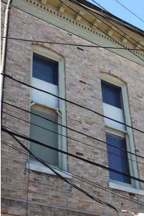
Figure 3.232, Wallace Library, East elevation, detail of first and second floor windows.
