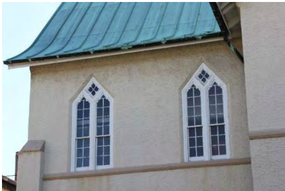
Figure 3.18, Historic Renwick Courthouse, north elevation, view of second-story windows at east end of elevation.
