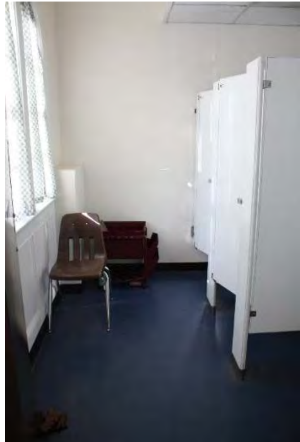
Figure 3.69, Historic Courthouse, First Floor, Room 116, general view looking west.
