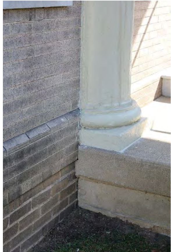
Figure 3.214, Wallace Library, West elevation, detail of foundation.
