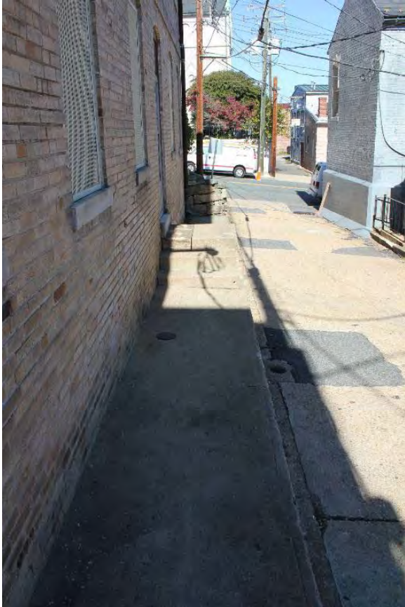
Figure 3.234, Wallace Library, East elevation, site, view to north.
