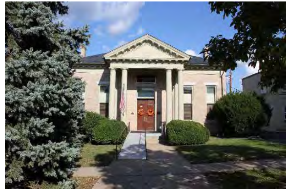
Figure 3.211, Wallace Library, West elevation, general view east.
