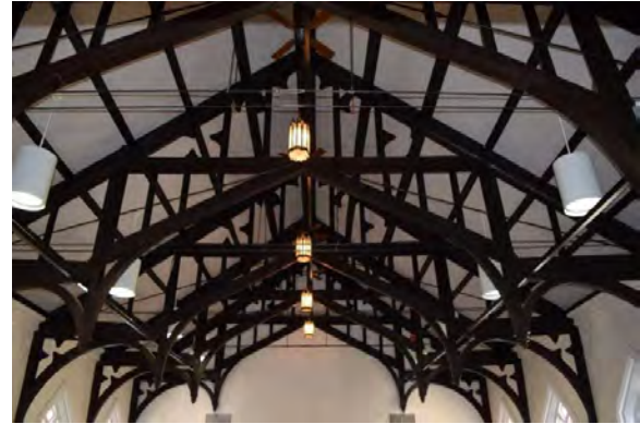
Figure 4.19: Hammer-bam trusses at courtroom roof
