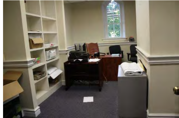
Figure 3.87, Historic Courthouse, First Floor, Room 122, general view looking west. Note the built-in shelves at the south wall, carpeted floor, and the higher level of detail including molded chair rail and base.
