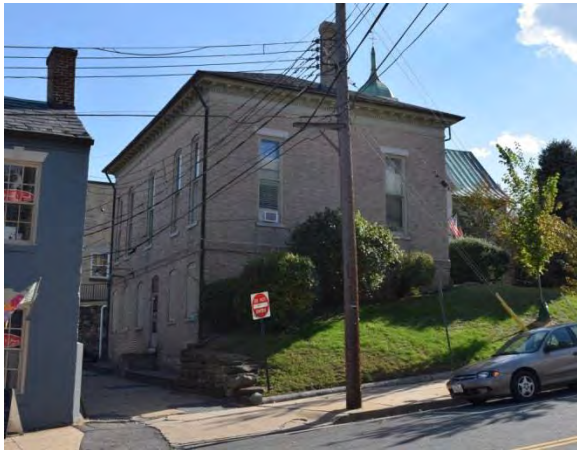
Figure 4.47: View of North and East Facades of the Wallace Library showing site grading
