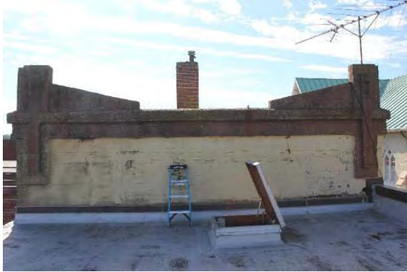
Figure 3.317, Old Jail, roof, view looking south toward higher roof.
