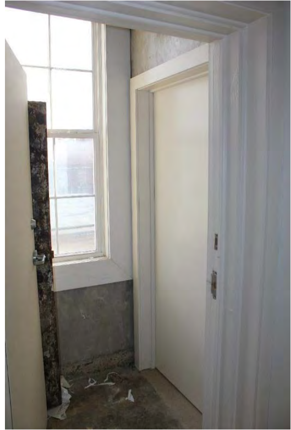
Figure 3.400, Old Jail, First Floor, Room 104, view of east vestibule.
