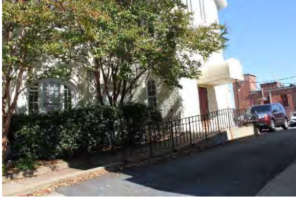
Figure 3.38, Historic Renwick Courthouse, south elevation, view of accessible ramp and entry.
