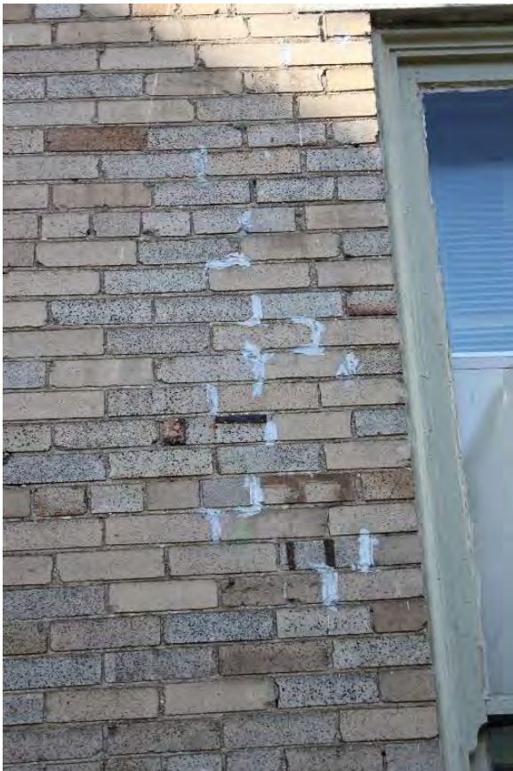
Figure 3.241, Wallace Library, South elevation, wall detail.
