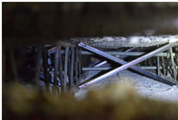
Figure 4.11: Open web steel joists at north wing attic
