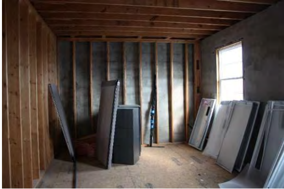
Figure 3.453, Old Jail, Second Floor, Room 202, general view looking north in the east end of the room.
