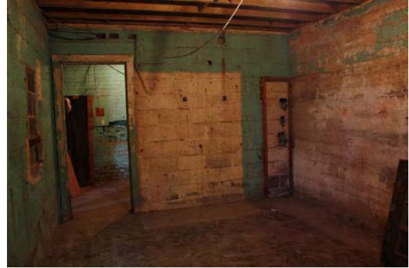
Figure 3.378, Old Jail, Basement, Room 005, general view looking south.
