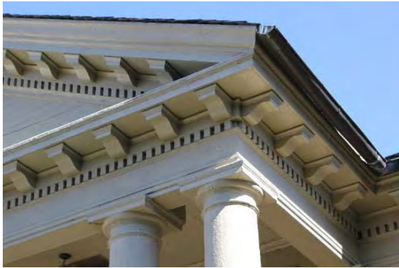
Figure 3.212, Wallace Library, West elevation, detail of cornice.
