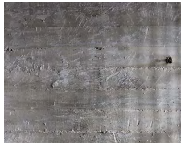
Figure 3.417, Old Jail, First Floor, Room 107, detail view of poured-in-place concrete wall.
