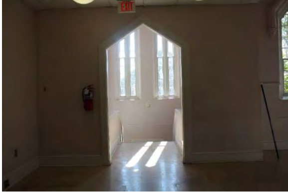
Figure 3.118, Historic Courthouse, Second Floor, Room 201, view of doorway leading to Stairway 1 (Room 101).
