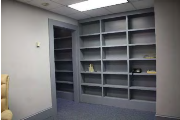
Figure 3.195, Historic Courthouse, Second Floor, Room 225, general view looking northeast.
