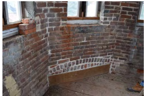
Figure 4.40: Base support of octagonal tower walls
