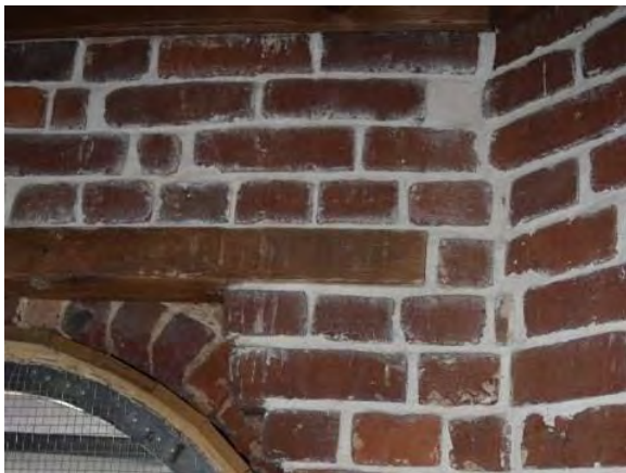
Figure 4.42: Repointing efforts at top of masonry tower
