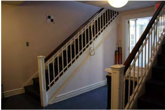
Figure 3.111, Historic Courthouse, First Floor, Room 132 (Stairway 2), general view of the staircase.
