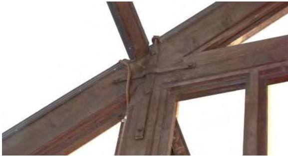
Figure 4.23: Top chord connection to collar tie and hammer post
