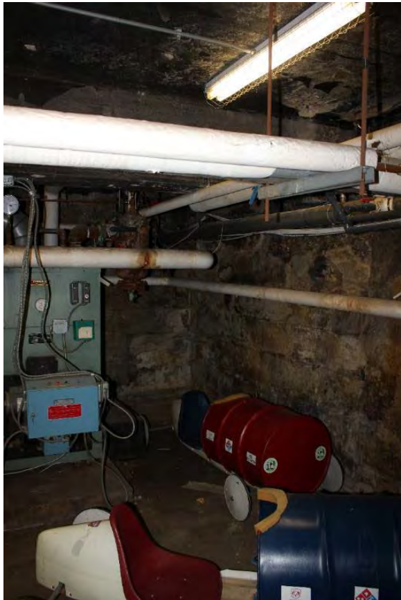
Figure 3.358, Old Jail, Basement, Room 002, general view looking south.
