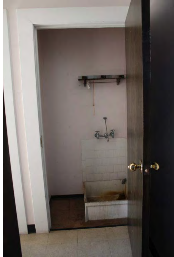
Figure 3.135, Historic Courthouse, Second Floor, Room 207, general view of room.
