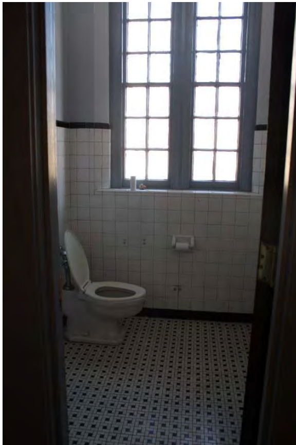
Figure 3.178, Historic Courthouse, Second Floor, Room 219, general view.
