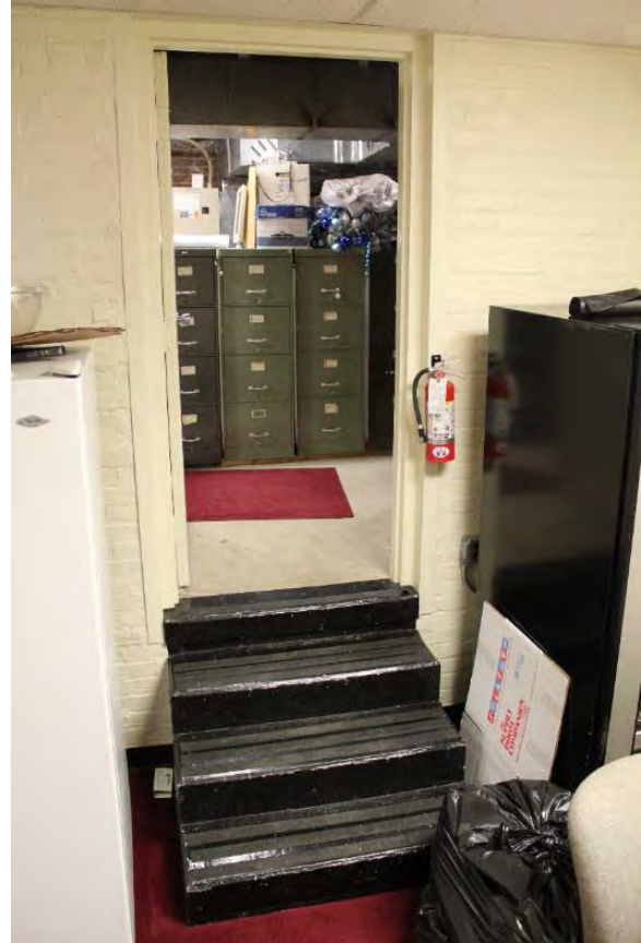
Figure 3.258, Old Wallace Library, Basement, Room 004, view of short flight of wood stairs and door leading to Room 001.
