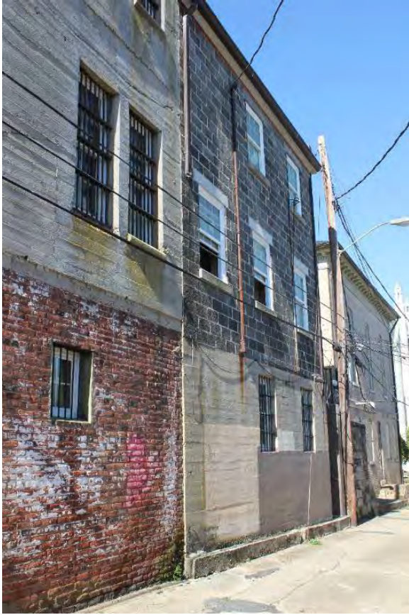
Figure 3.335, Old Jail, east elevation, general view of north end.
