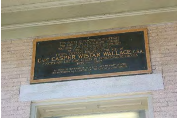
Figure 3.220, Wallace Library, West elevation, detail of dedication plaque.
