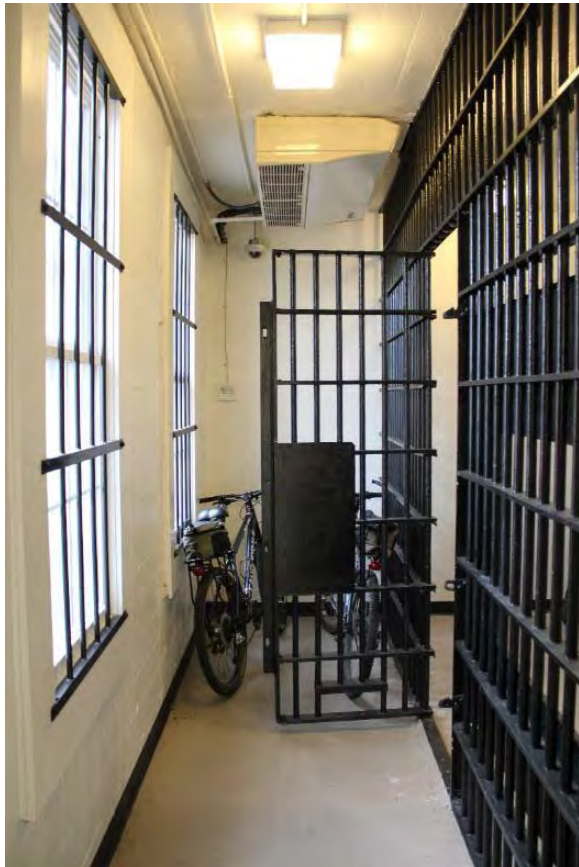
Figure 3.384, Old Jail, First Floor, Room 101, general view looking south at the east end of the room. Note the iron bars for the jail cell at the west end of the room.
