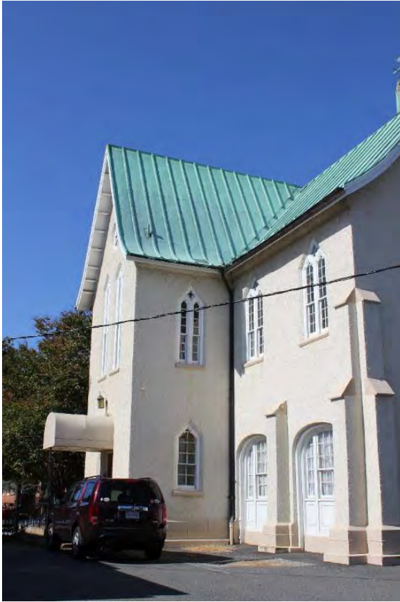
Figure 3.31, Historic Renwick Courthouse, south elevation, general view.
