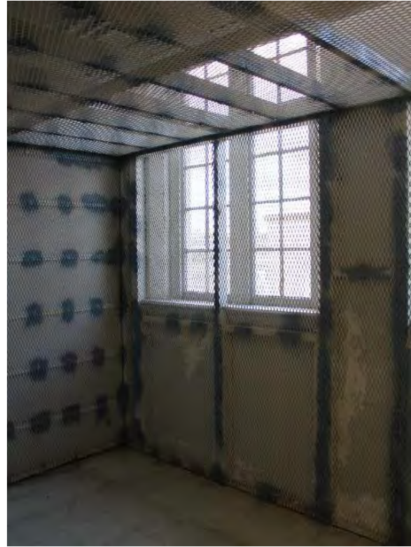
Figure 3.187, Historic Courthouse, Second Floor, Room 222, general view looking northeast.
