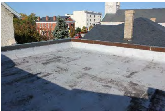
Figure 3.318, Old Jail, roof, view looking northwest over lower, sloped membrane roof.
