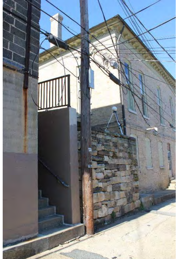
Figure 3.235, Wallace Library, East elevation, site, view to northwest.
