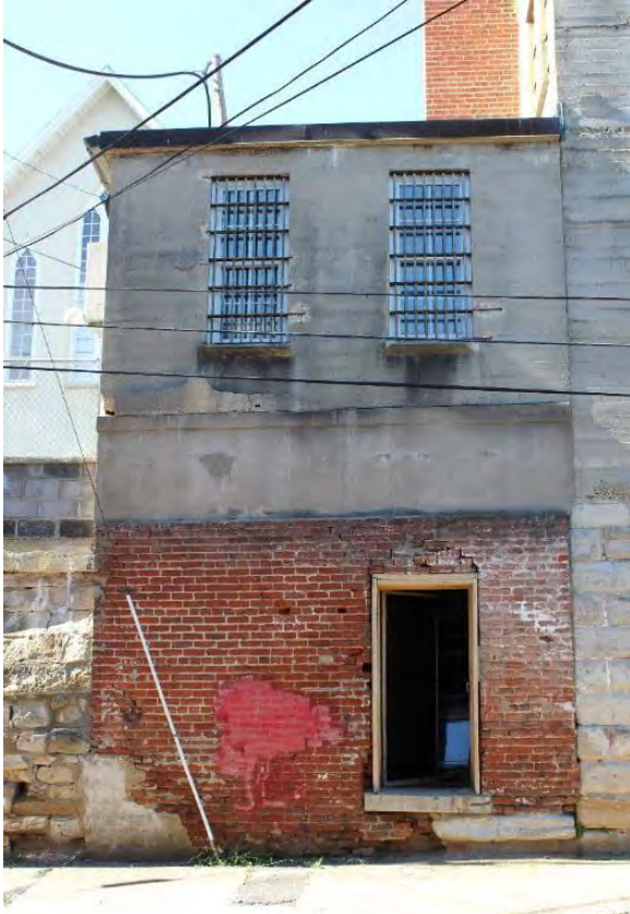
Figure 3.337, Old Jail, east elevation, general view of one-story wing at south end.
