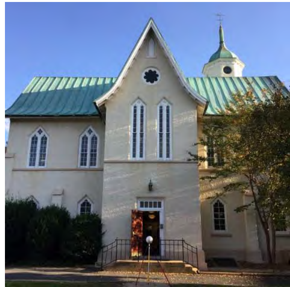
Figure 4.06: North courthouse elevation with projecting water-table.
