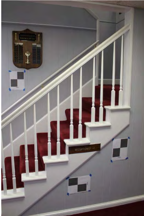
Figure 3.274, Old Wallace Library, First Floor, Room 104, view of wood balustrade.
