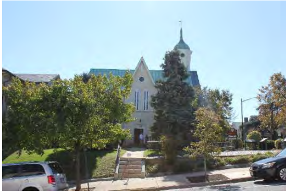
Figure 3.13, Historic Renwick Courthouse, north elevation, general view looking south.
