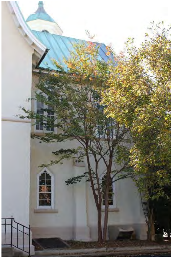
Figure 3.16, Historic Renwick Courthouse, north elevation, view of west end of elevation.
