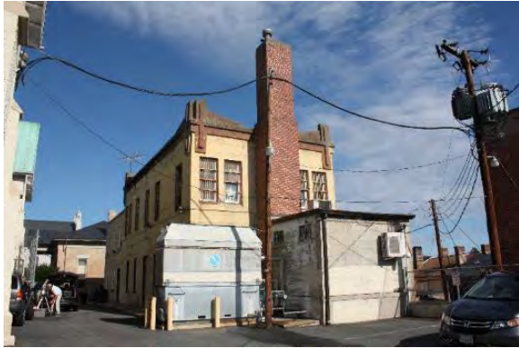
Figure 3.348, Old Jail, south elevation, general view looking north.
