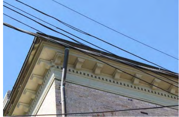
Figure 3.229, Wallace Library, East elevation, cornice detail.
