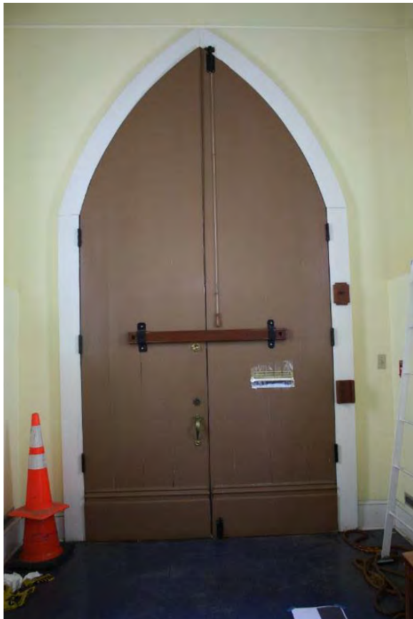
Figure 3.81, Historic Courthouse, First Floor, Room 119, view of main entry doors at west wall.
