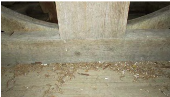
Figure 13: Bell support truss pegged mortise and tenon connections
