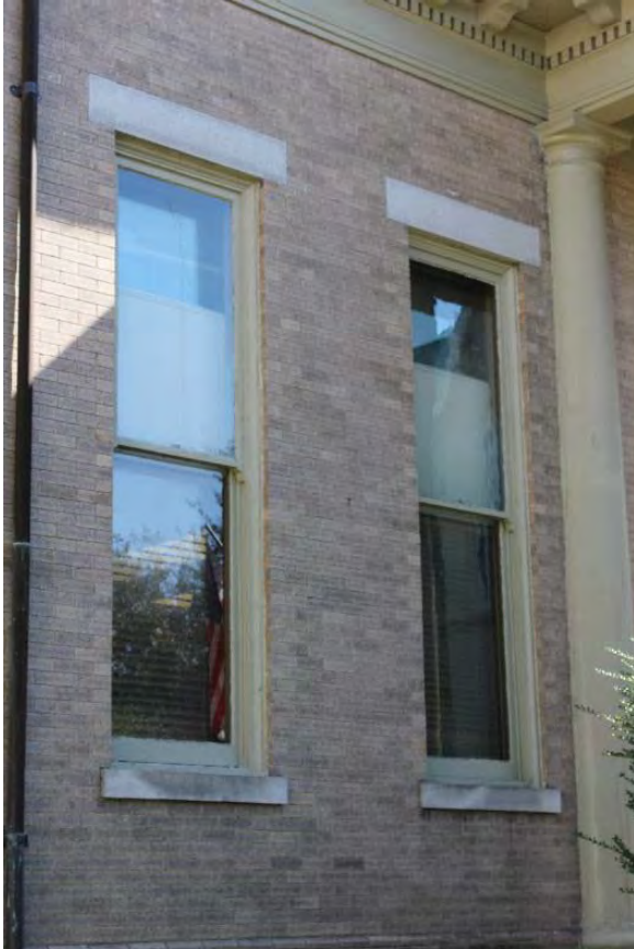
Figure 3.215, Wallace Library, West elevation, detail of windows. Note the second floor structure visible through the windows. Note the staining on the stone sills.
