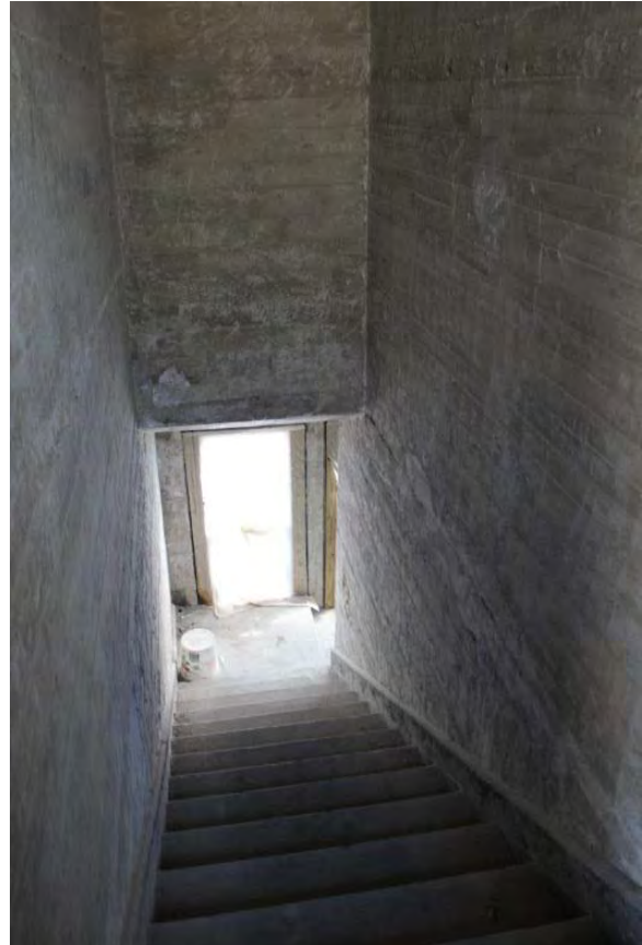
Figure 3.423, Old Jail, First Floor, Room 108, view of stair from second story.
