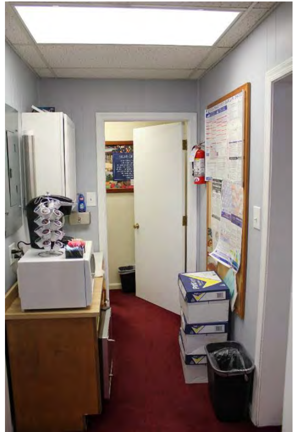
Figure 3.285, Old Wallace Library, First Floor, Room 108, general view looking south.
