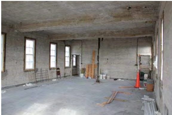
Figure 3.438, Old Jail, Second Floor, Room 201, view looking northwest.
