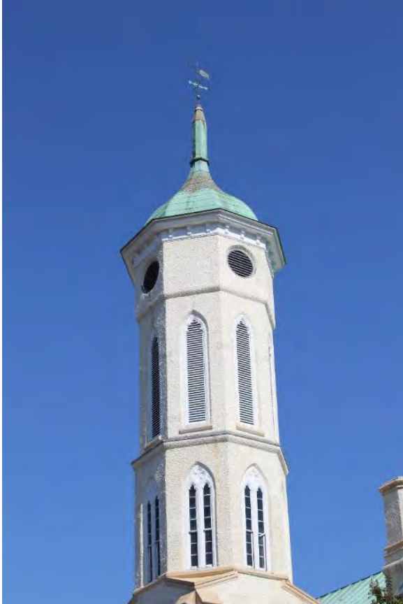
Figure 3.5, Historic Renwick Courthouse, west elevation, view of upper stories of bell tower.
