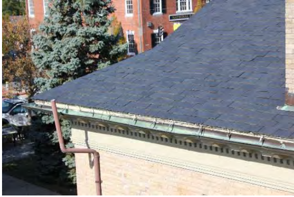
Figure 3.240, Wallace Library, South elevation, cornice detail.
