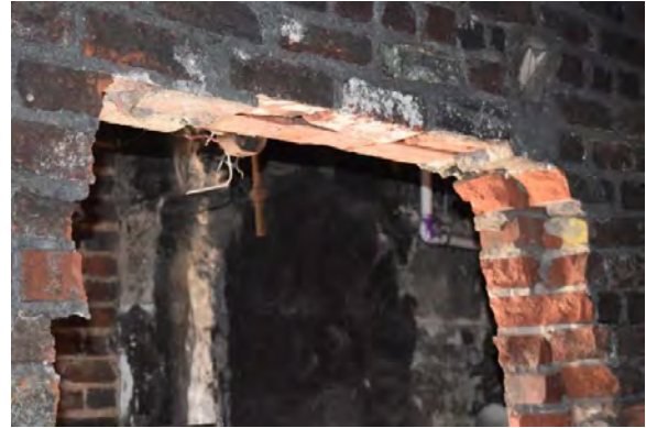
Figure 4.73: Unsupported masonry in center basement
