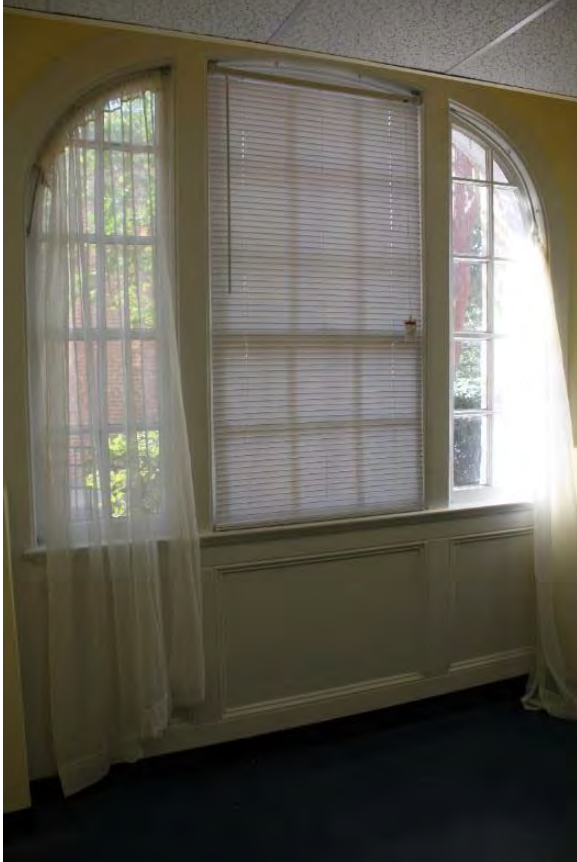
Figure 3.54, Historic Courthouse, First Floor, Room 105, view of arched window.
