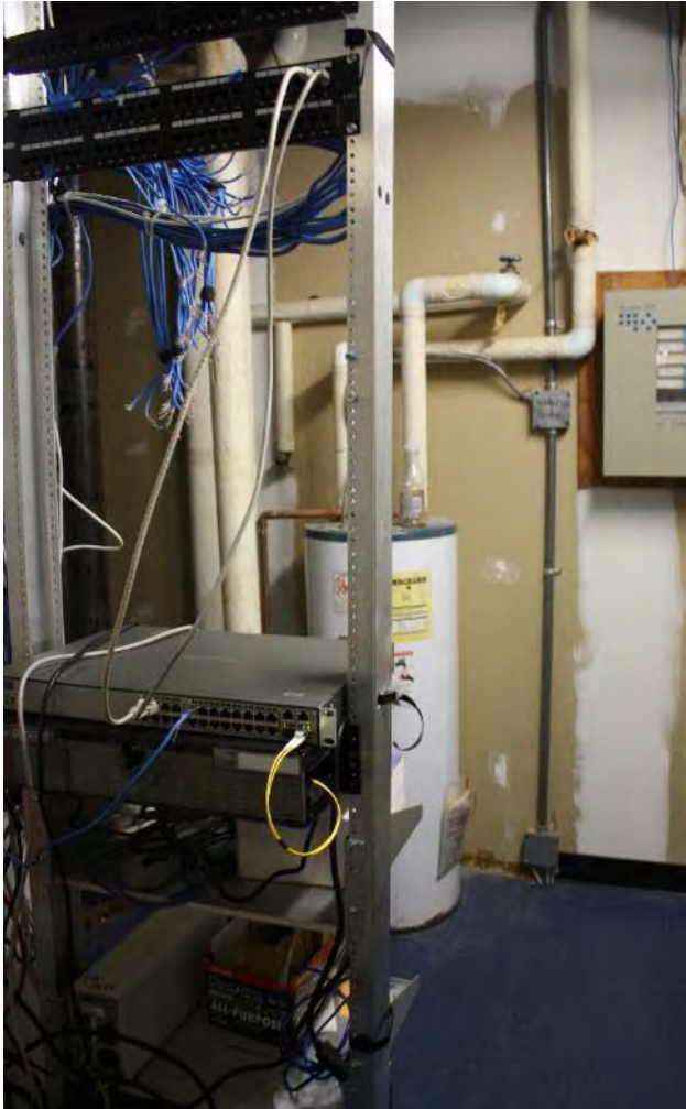
Figure 3.59, Historic Courthouse, First Floor, Room 108, general view.
