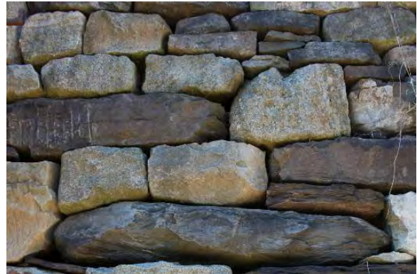
Figure 3.236, Wallace Library, East elevation, detail of stone retaining wall.
