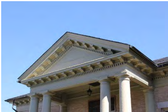
Figure 3.213, Wallace Library, West elevation, detail of porch roof.
