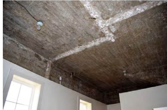
Figure 4.80: Location of removed concrete wall in cast-in-place concrete jail house
