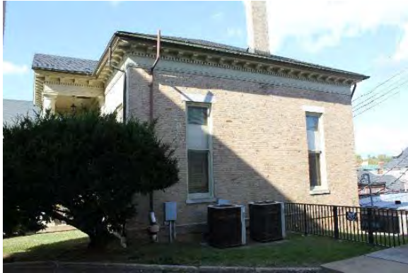
Figure 3.237, Wallace Library, South elevation, view northeast.
