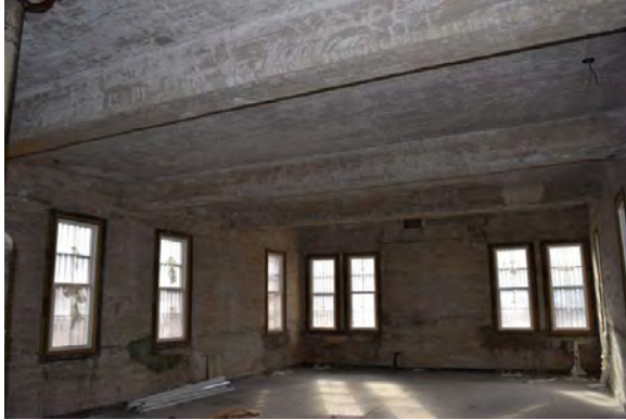
Figure 4.81: Center building second floor space with cast-in-place roof structure above
