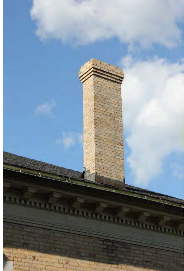
Figure 3.238, Wallace Library, South elevation, detail of chimney.
