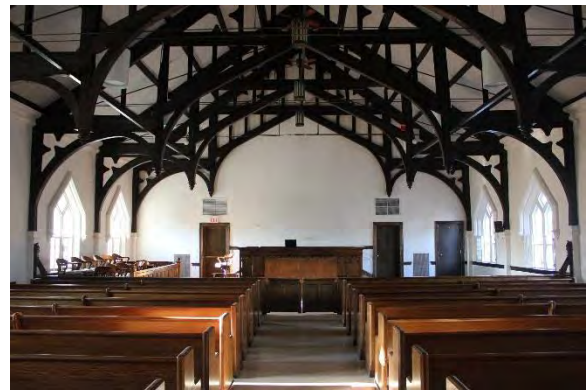
Figure 2.40, Fredericksburg Courthouse, Courtroom showing second floor, inserted in 1948, view to north, 2015.
