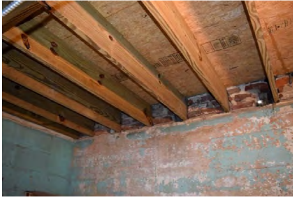
Figure 4.79: Northern addition first floor joists bearing on perimeter concrete wall
