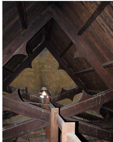
Figure 4.28: Ornate scissor roof trusses in south wing
