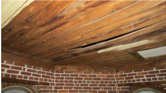
Figure 3: 5 th Floor Ceiling
