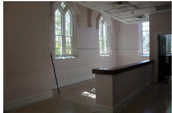
Figure 3.120, Historic Courthouse, Second Floor, Room 202, general view looking southwest. Note the low dividing north wall.
