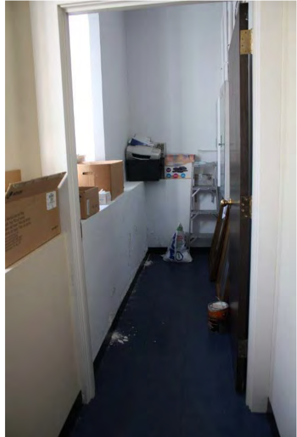
Figure 3.104, Historic Courthouse, First Floor, Room 128, general view of room looking south. Note the built-in ledge at the walls.
