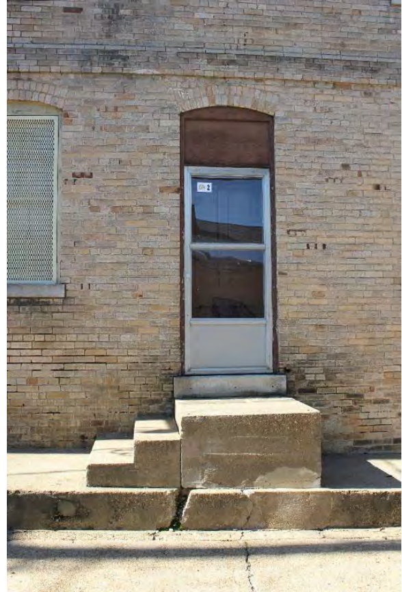
Figure 3.233, Wallace Library, East elevation, basement door and concrete stoop detail.
