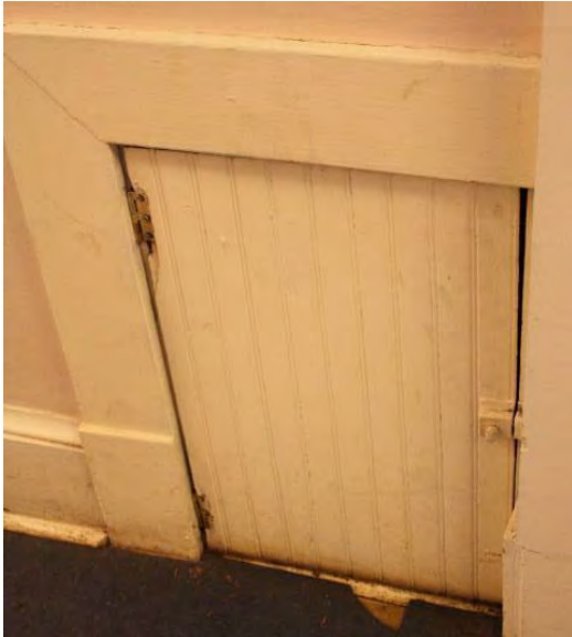
Figure 3.44, Historic Courthouse, Stair Landing, Room 101, view of small door under stair.
