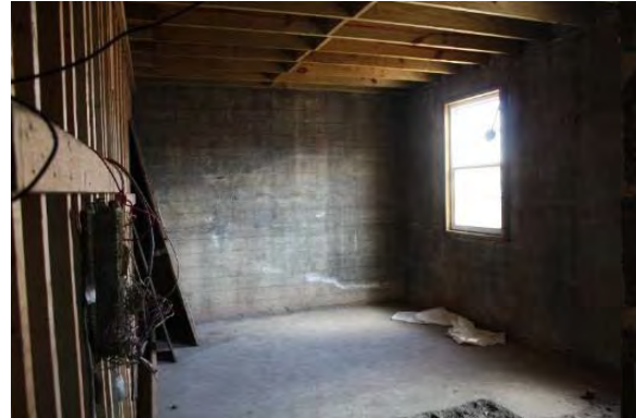
Figure 3.381, Old Jail, Basement, Room 006, general view looking northeast.
