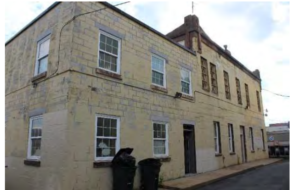
Figure 3.316, Old Jail, west elevation, general view looking southeast.
