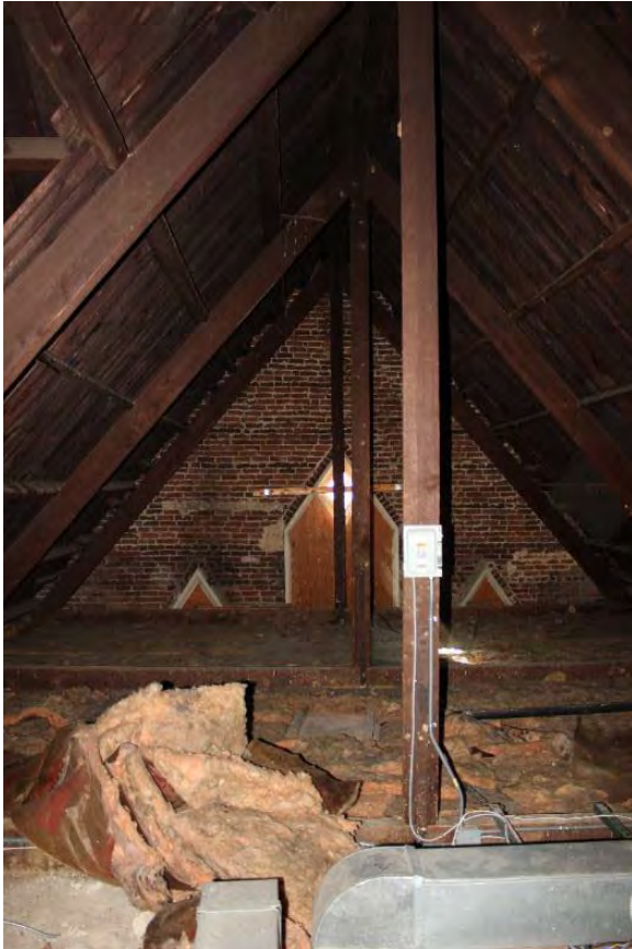
Figure 3.206, Historic Courthouse, North Attic, Room 303, general view looking west.
