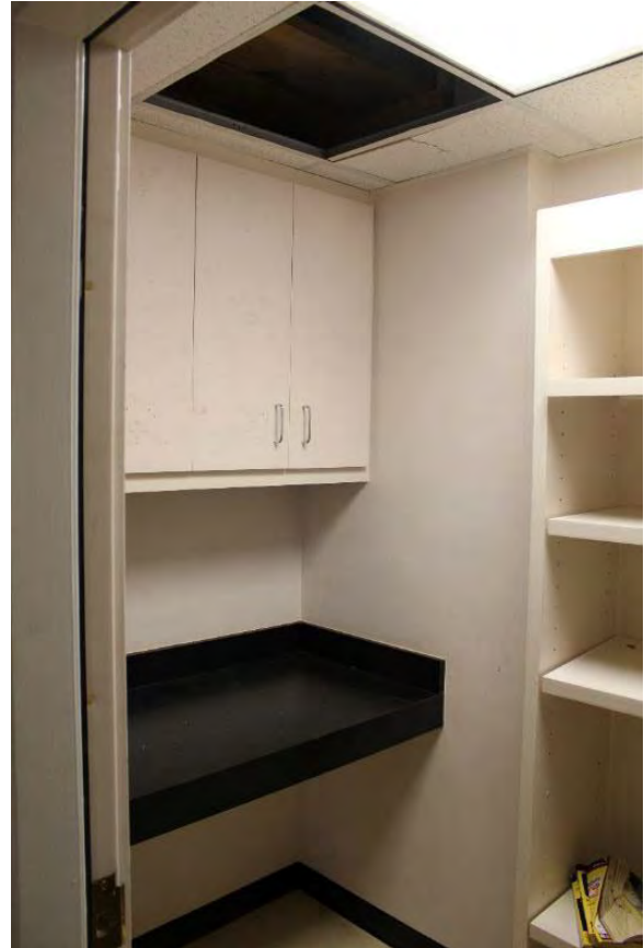
Figure 3.196, Historic Courthouse, Second Floor, Room 226, general view. Note the missing ceiling tile and adjacent cracked tile.
