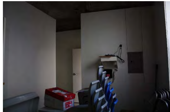
Figure 3.406, Old Jail, First Floor, Room 105, general view looking south.
