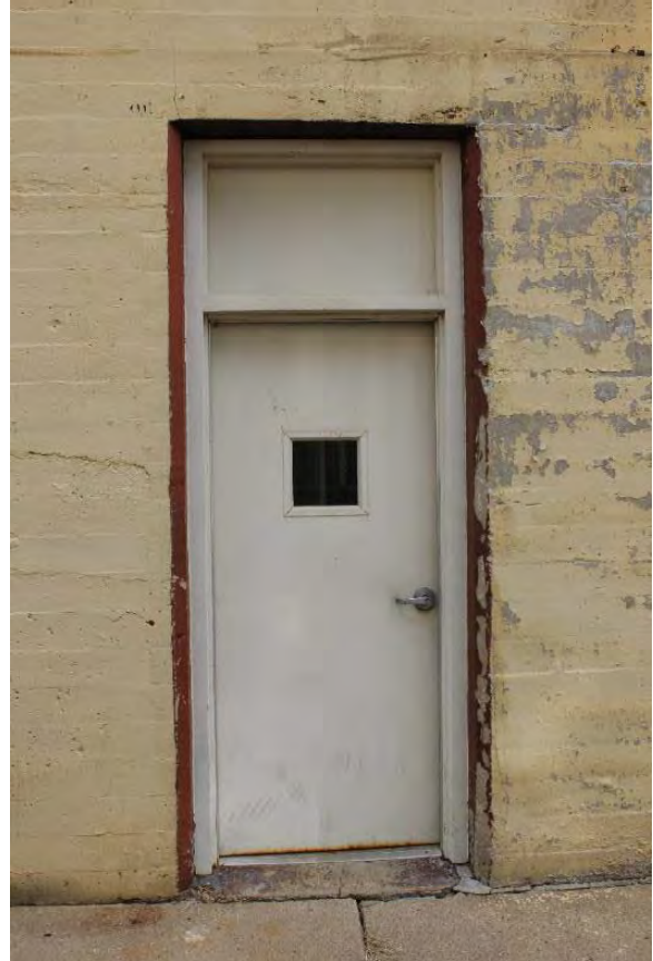
Figure 3.329, Old Jail, west elevation, view of south door.
