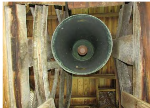
Figure 5: Underside of bell from floor below
