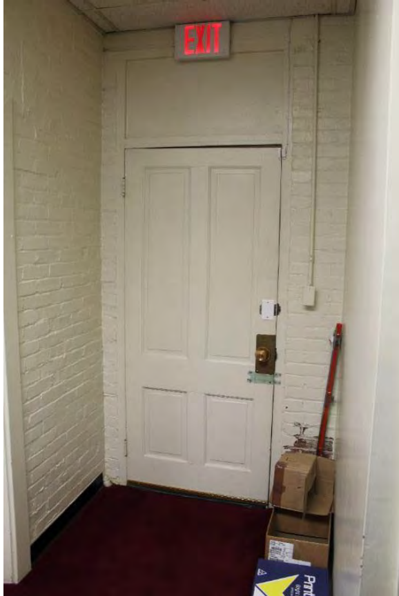
Figure 3.257, Old Wallace Library, Basement, Room 004, view of the early-twentieth-century, wood, four-panel exterior door at east wall.
