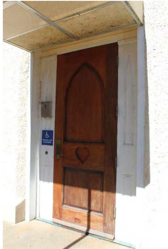
Figure 3.37, Historic Renwick Courthouse, south elevation, view of door at accessible entry.
