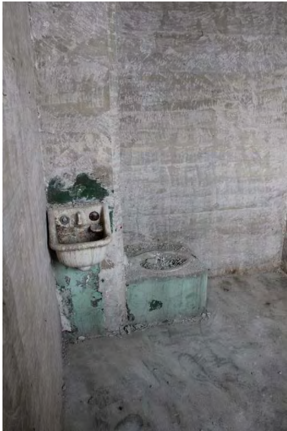
Figure 3.415, Old Jail, First Floor, Room 107, general view looking west.
