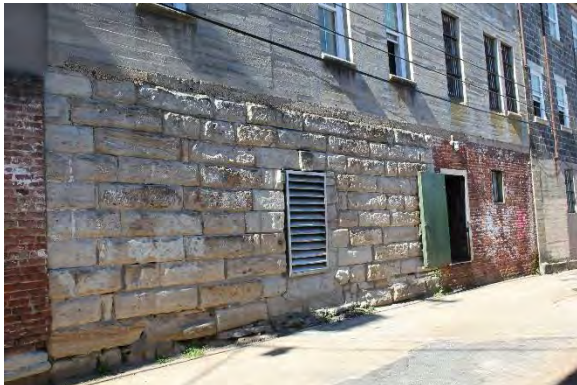
Figure 1.19, Old Jail. Visible layers of history: early stone, later brick, and the existing concrete jail. Photograph 2015.
