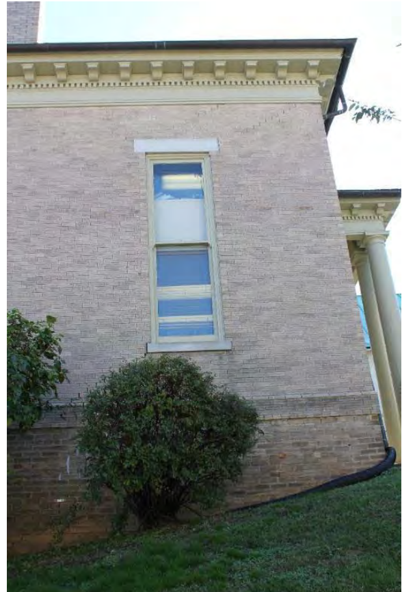
Figure 3.226, Wallace Library, North elevation, detail of window.
