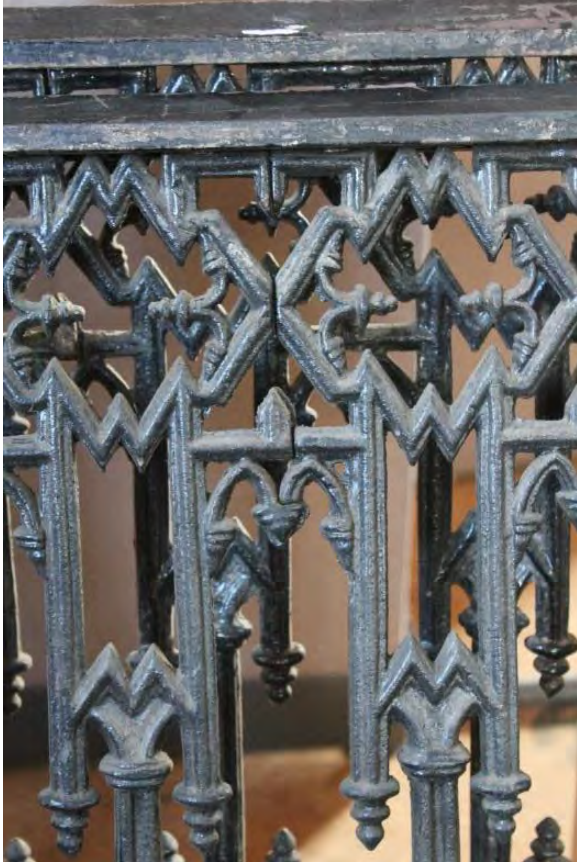
Figure 3.457, Old Jail, Second Floor, Room 202, detail view of iron railing.
