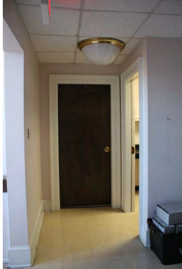
Figure 3.177, Historic Courthouse, Second Floor, Room 218, general view looking east.
