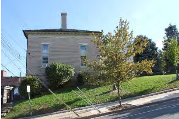
Figure 3.222, Wallace Library, North elevation, view south.
