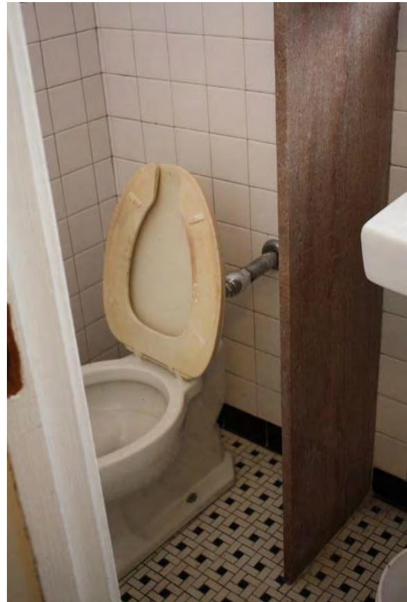
Figure 3.52, Historic Courthouse, First Floor, Room 104, general view of the room.
