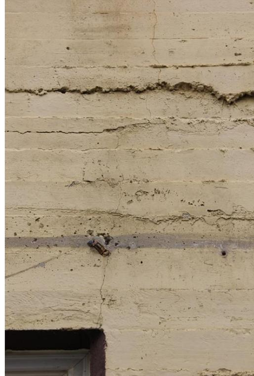
Figure 1.16, Old Jail. Cracking of the exterior concrete wall surfaces. Photograph 2015.
