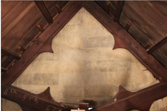
Figure 1.5, Fredericksburg Courthouse, South attic. Evidence of the original surface treatment of the exterior (which survives on the portion of the South attic above the early 20<sup>th</sup> century ceiling) remains, as does the interior finish itself. Photograph 2015.
