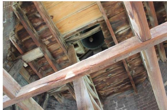
Figure 1.4, Fredericksburg Courthouse, bell tower. Moisture infiltration into the bell tower. Photograph 2015.
