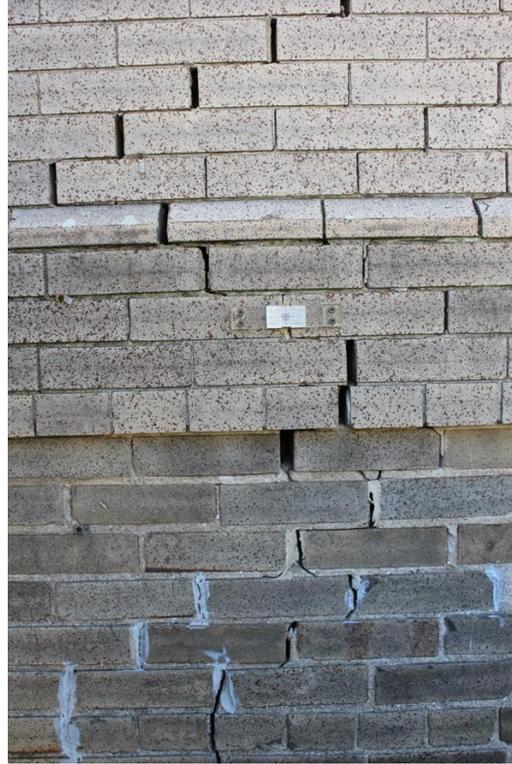
Figure 1.11, Wallace Library. Pervasive shifting and cracking of brick in the north elevation. Photograph 2015.
