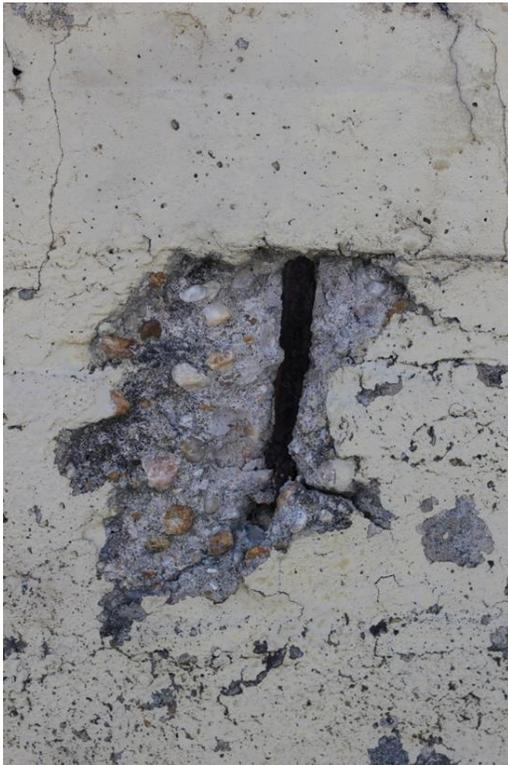
Figure 1.15, Old Jail. Rust-jacking and spalling of the exterior concrete wall surfaces. Photograph 2015.
