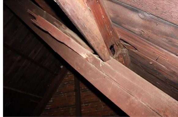
Figure 1.2, Fredericksburg Courthouse, North attic. Shifting of and damage to structural members. Photograph 2015.
