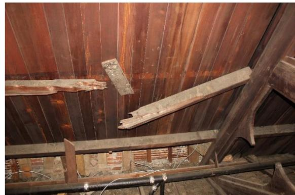
Figure 1.3, Fredericksburg Courthouse, North attic. Broken truss. Photograph 2015.
