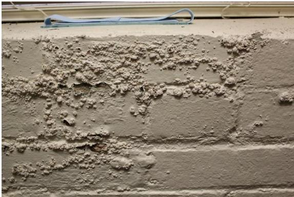
Figure 1.10, Wallace Library. Persistent moisture infiltration in the basement. Photograph 2015.
