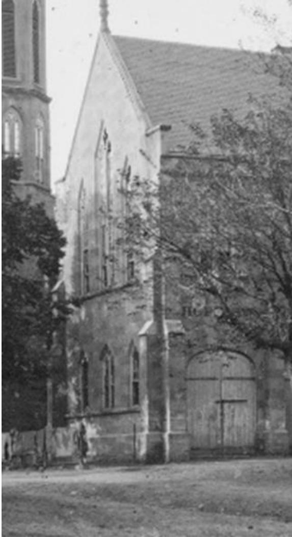
Figure 1.7, Fredericksburg Courthouse, South Wing. Image of the original parapets and roof slope, removed by later alterations. Photograph 1865.
