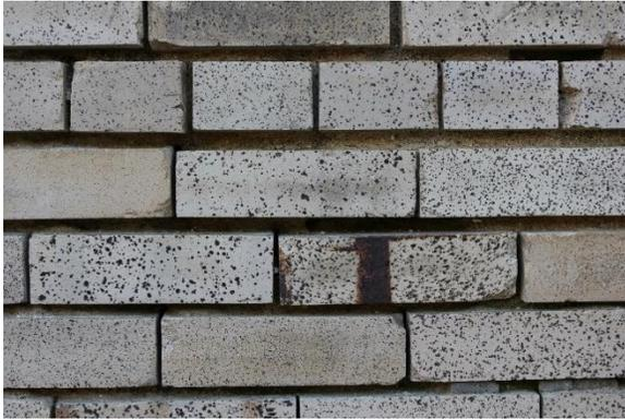
Figure 1.9, Wallace Library. Extensive mortar loss in the north elevation. Photograph 2015.
