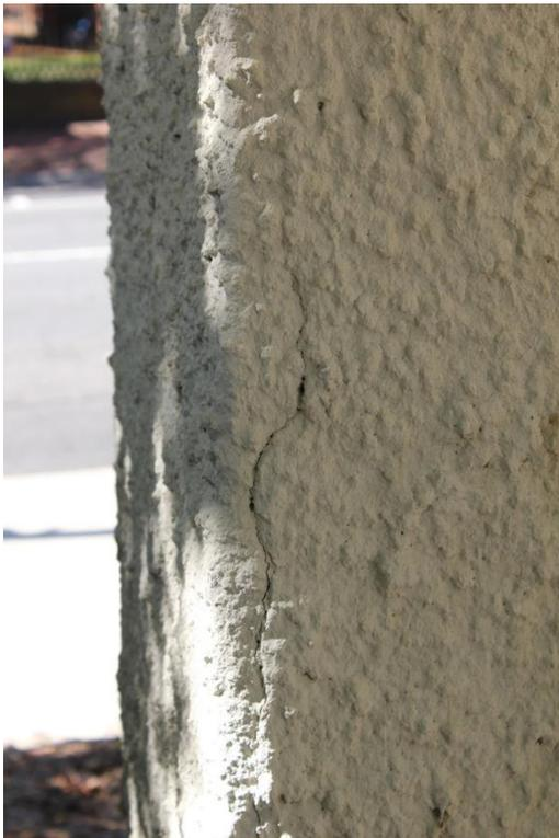
Figure 1.1, Renwick Courthouse, detail of exterior stucco. Note hairline cracks that result in moisture infiltration. Photograph 2015.
