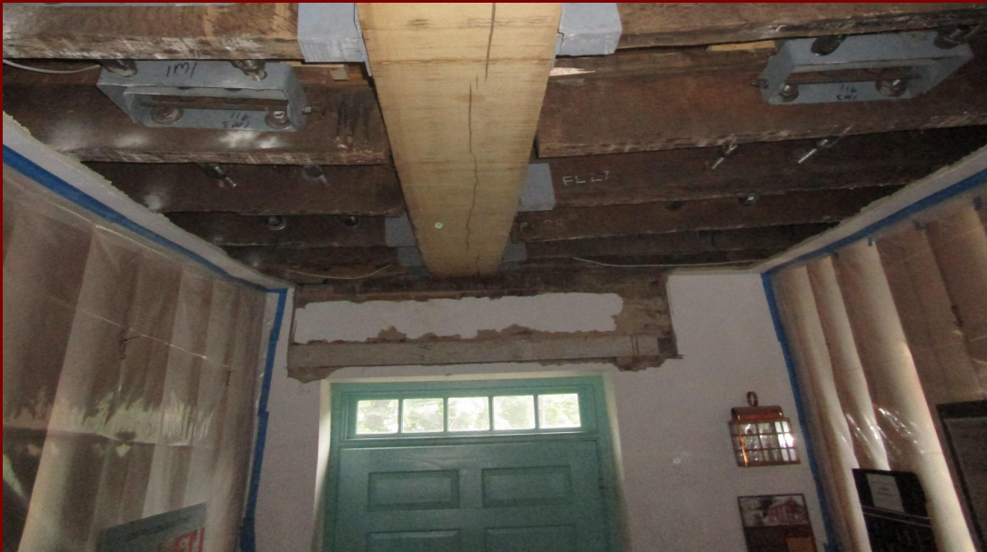
The sales room with its new summer beam, after this portion of the original beam failed.
