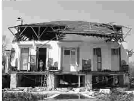
Jefferson Davis' home 'Belvoir' in Biloxi after Hurricane Katrina..
